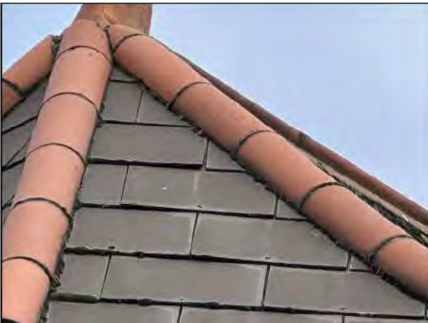
13 - Example of the lifting slates
