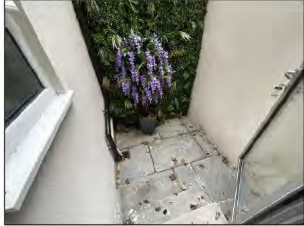
39 - Overview of the rear courtyard garden
