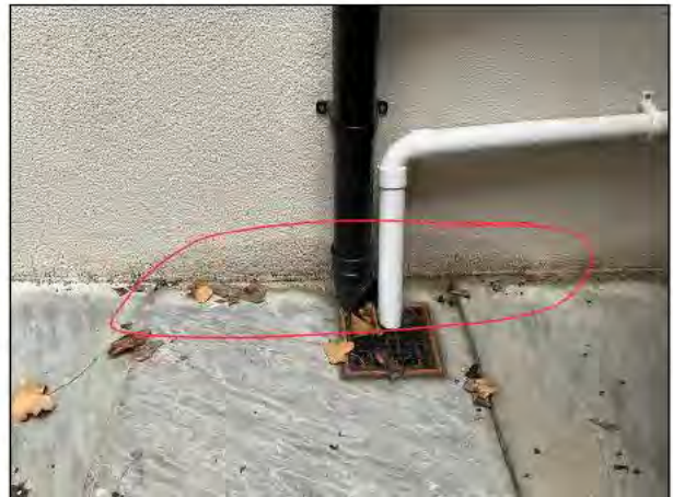
25 - Render in contact with the ground
