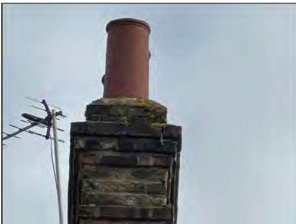
6 - Flashing and pots
