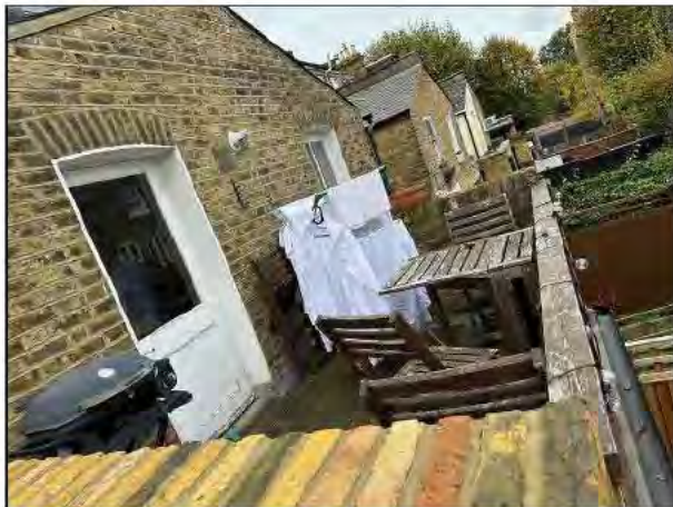
17 - Neighbours roof terrace
